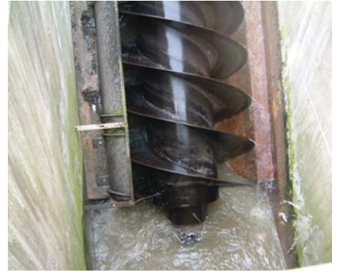
Archimedean screw fitted with AESSEAL® bearing seals in 2003 (Case Ref: 1348).
